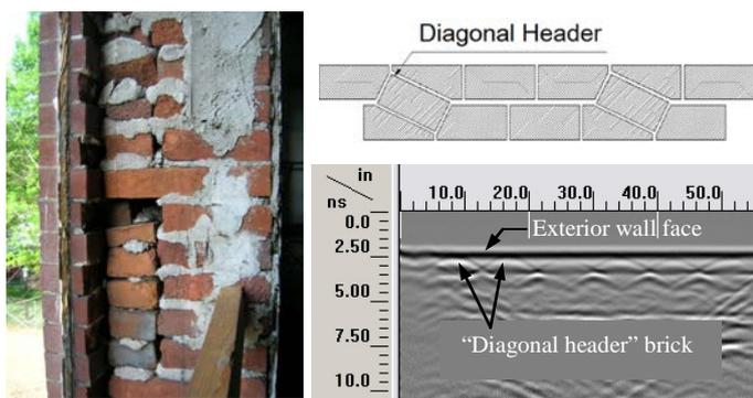
Fig. 2 Walls were built of poor quality construction (left) with many internal voids. Surface penetrating radar was used to locate voids and also identify hidden header locations. Hidden “diagonal” headers were missing at many locations, requiring remedial tie installation. The radar trace at lower right shows strong reflections at each header brick location.
